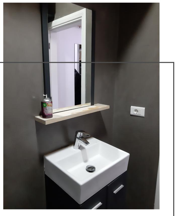
Microtopping wall is a single component thin concrete overlay
